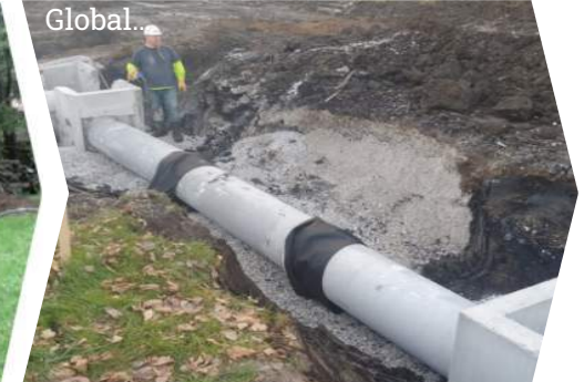
Image source: https://www.snyder-associates.com/projects/storm-water-drainage-improvements/
