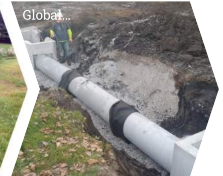
Image source: https://www.snyder-associates.com/projects/stormwater-drainage-improvements/
