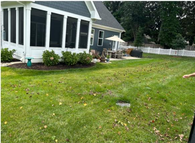
Poor Grading leads to water flooding this backyard
