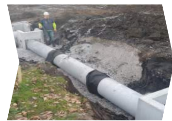
Image source: https://www.snyder-associates.com/projects/stormwater-drainage-improvements/
