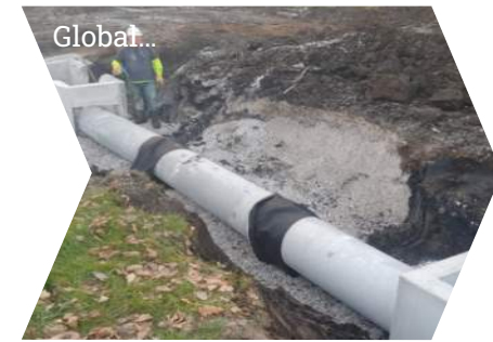
Image source: https://www.snyder-associates.com/projects/stormwater-drainage-improvements/
