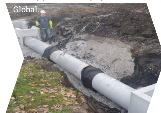
Image source: https://www.snyder-associates.com/projects/stormwater-drainage-improvements/
