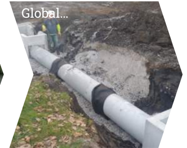
Image source: https://www.snyder-associates.com/projects/stormwater-drainage-improvements/
